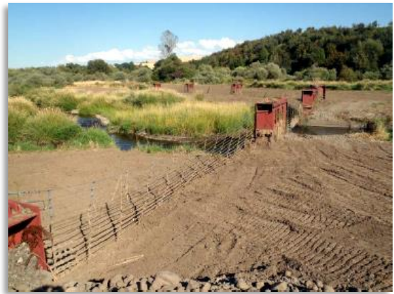
FIGURE 10: FOREBAY DEBRIS BARRIER. LOOKING SOUTHEAST AFTER VEGETATION CLEANING IN AUGUST 2011 (USACE image)
