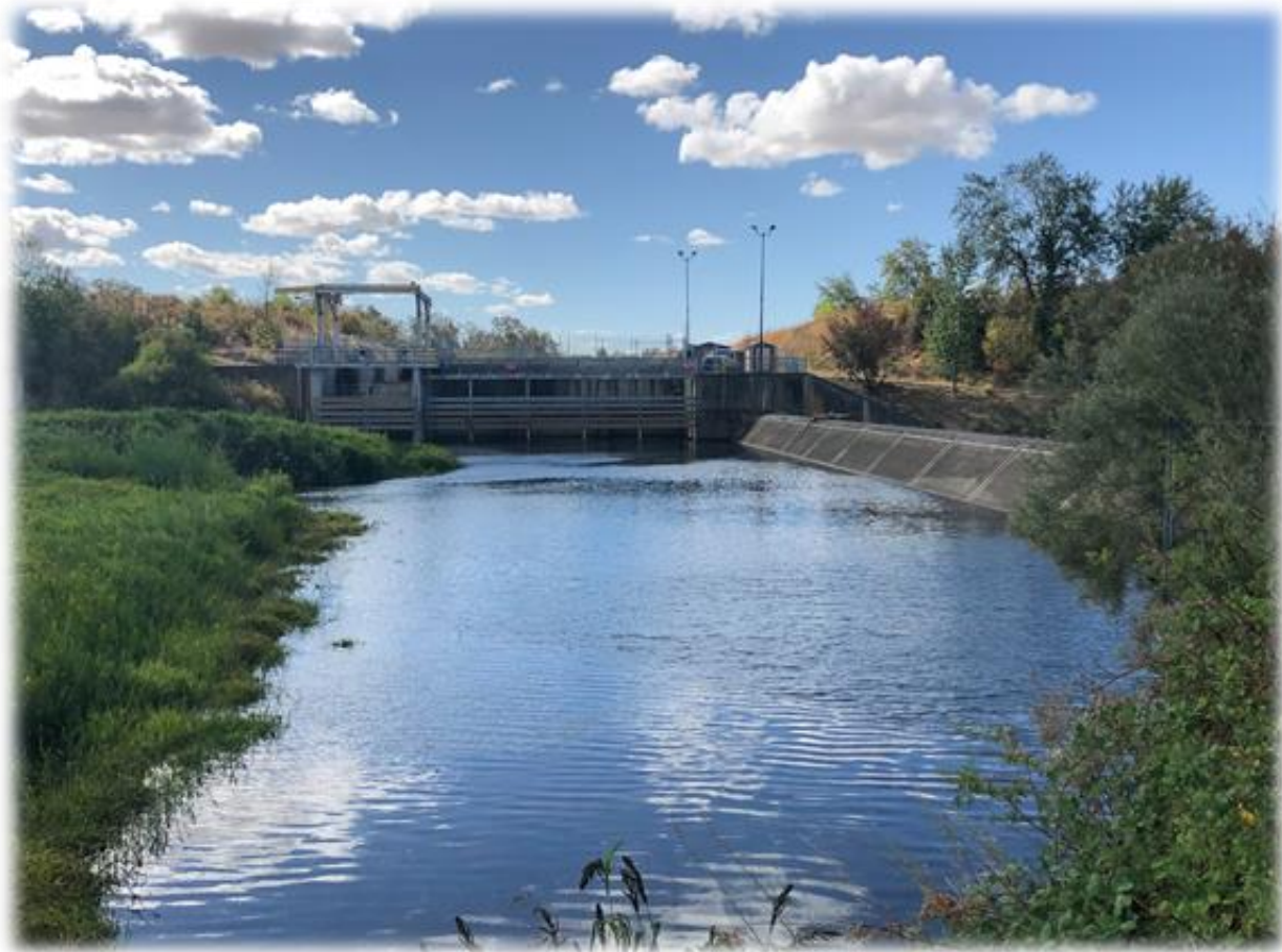
IMAGE 3: VIEW OF DIVERSION DAM AND SPILLWAY FROM RIGHT BANK OF MILL CREEK. SEPTEMBER 2021 (USACE image)
